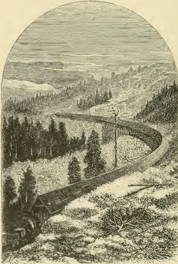
SNOW SHEDS ACROSS THE SIERRAS.
