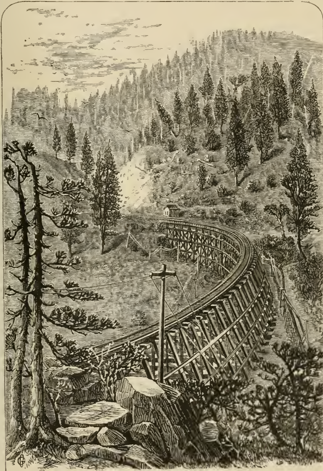
SECRET TOWN, TRESTLE-WORK.
