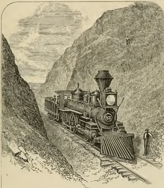
ROCK CUT, NEAR ASPEN.
