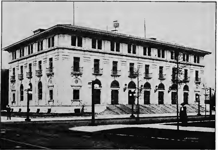
WIDE RANGE OF POST OFFICE BUILDINGS
