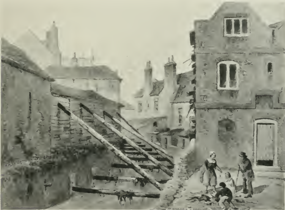
FLEET DITCH, WEST STREET, SMITHFIELD, AS IT WAS IN 1844
