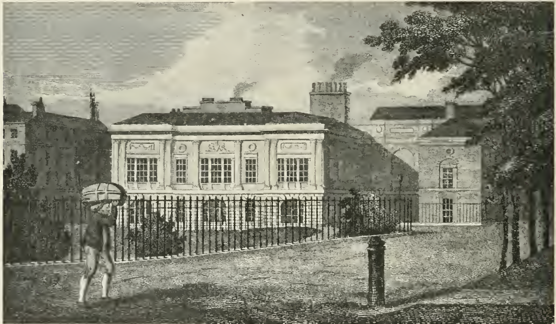
TRINITY HOUSE, TOWER HILL
