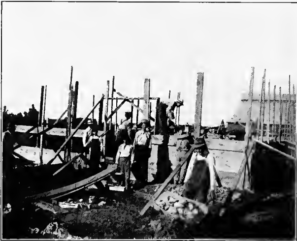
STUDENTS CONSTRUCTING A CONCRETE FOUNDATION FOR A BARN.
