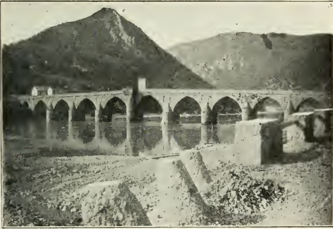
OLD BRIDGE AT VIŠEGRAD. (From a Photo, by Miss Chadwick.)
