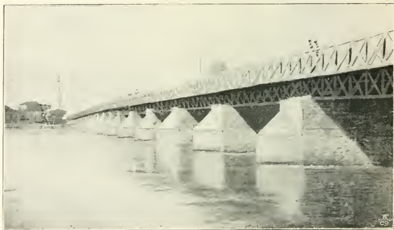
BRIDGE OVER THE MARICA, SCENE OF THE PHILIPPOLIS MURDER. (From a Photo. by Mr. Wratistaw.)
