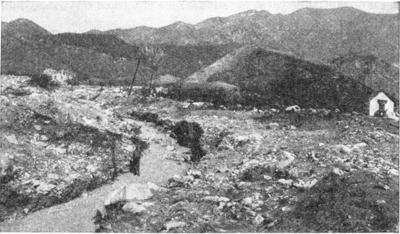
FIGURE 34.—Dunsmere Creek, ravaged by flood from the burned area. Line of boulders near the building indicates extent and force of the torrent. All trees were torn from the stream banks, and rock-mattress check dams were swept from its bed. Man stands near the remains of one of the wire-bound dams. Compare with figure 35.
