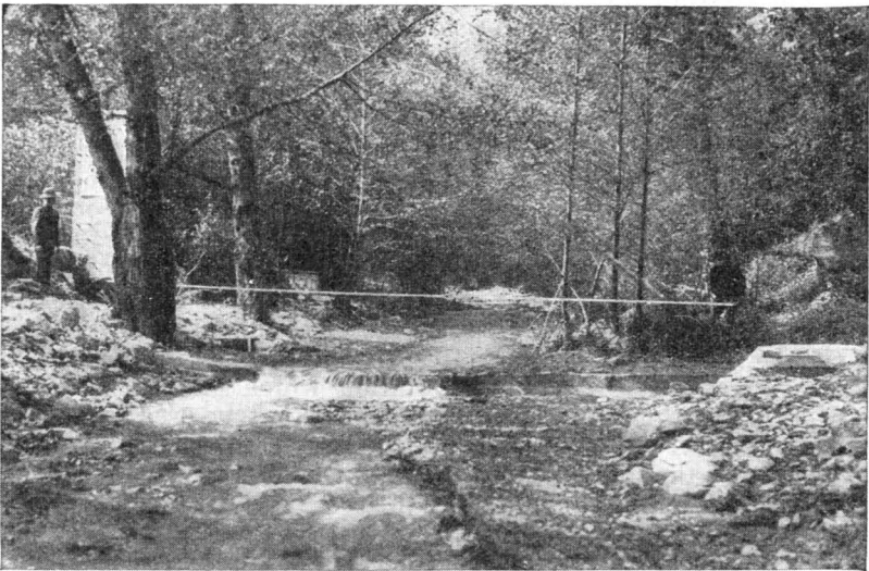
FIGURE 35.—Arroyo Seco Creek, undamaged by storm run-off from forest-covered watershed adjacent to the burned area. White line shows high-water mark of the New Year's storm. The water, being clear and controlled, was harmless. Compare with figure 34.
