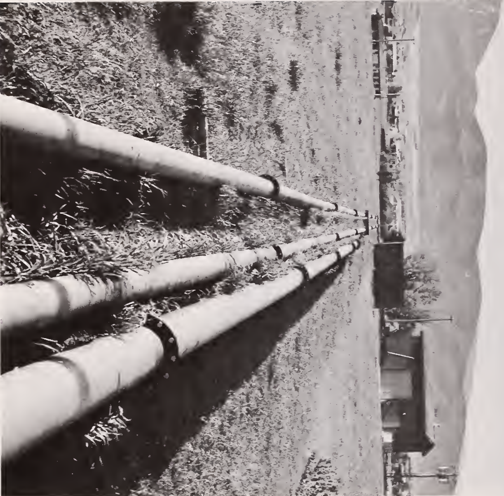
Prototype hydraulic wood chip pipeline.
