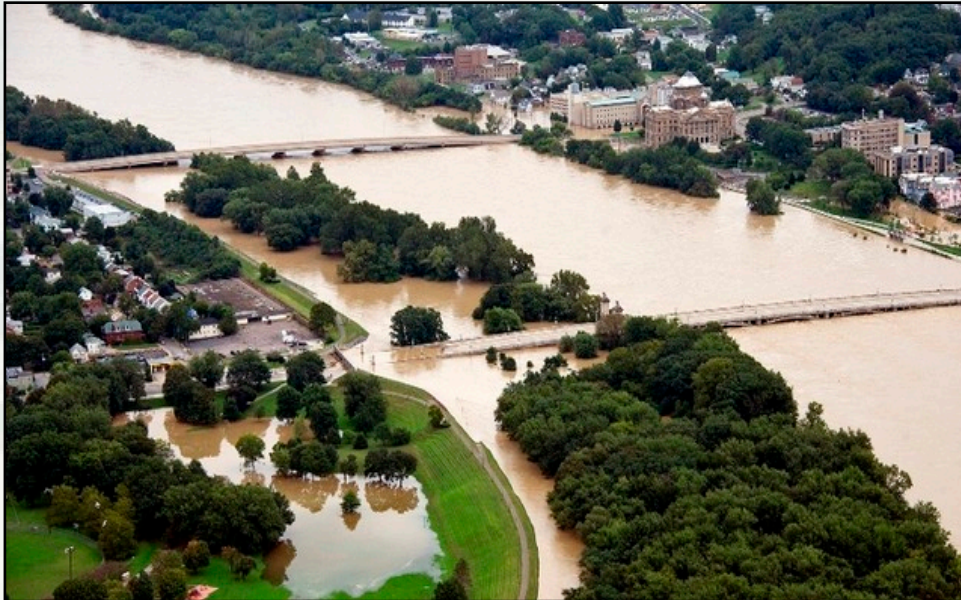
Wilkes Barre, PA – Pierce & Market Street Bridges
