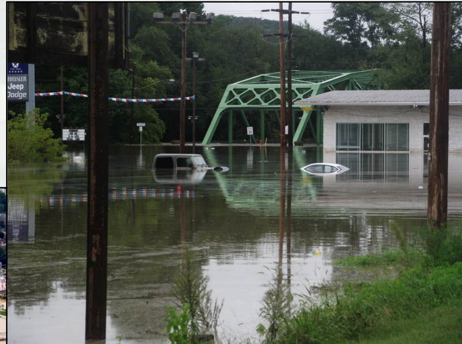
Sunbury, PA – Rt. 61 Bridge
