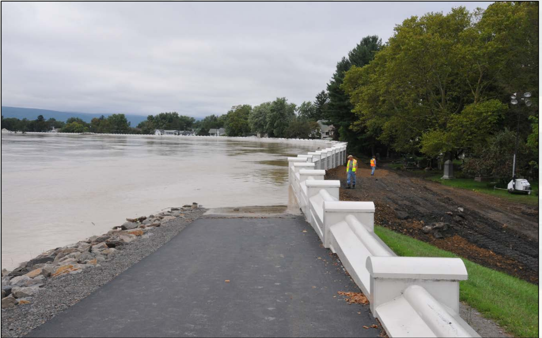
Wyoming Valley, PA – Reinforcement on Landside of Wall
