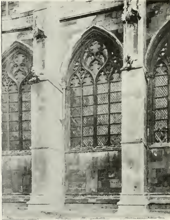
F. B. Beverley Minster : North Nave
