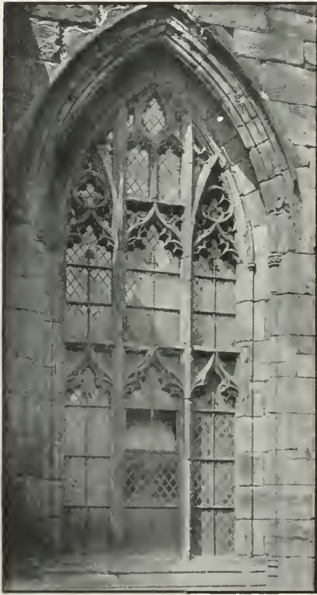
F. H. C. Nantwich, Cheshire: North Transept
