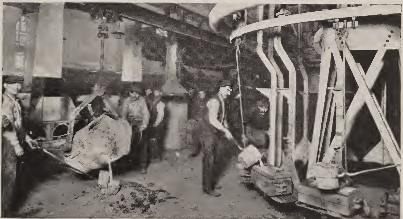
Rehandling is saved (upper left) by chuting material from machine to machine; by testing gasoline engines on a truck (upper right), (A) safety covering over shaft projection, (B) tongue, (C) wedge; and by bench-high trucks (middle left). Special trucks give "fewer motions" in handling bath tubs (middle right). In the Ford foundry a "merry-go-round" conveyor brings the molds to the men
