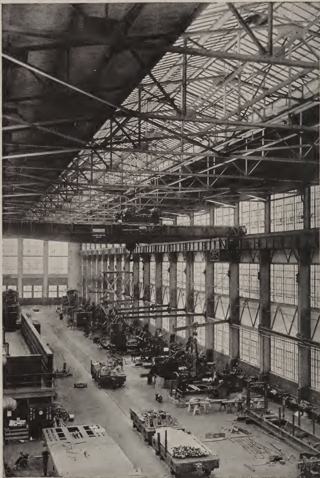
M ACHINERY and equipment function better when the building has been constructed around them, as in the Industrial Works at Bay City, Michigan. In the erection department, the side-wall columns carry jib-cranes for local material handling. Above travels a beam crane for complete assemblies. An industrial railway brings in the parts and removes finished machines
