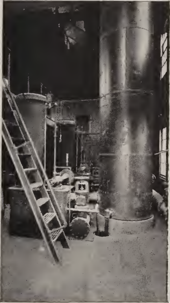
Internally-fired, horizontal boilers are compact and take little headroom (in middle, above); externally-fired boilers (on either side, above) stand higher, but give longer travel of the gases. Vertical boilers (right, below) require ample head-room, but are space-saving. Producer-gas furnaces (left, at American Graphophone Company) are space-saving, but require a high roof
