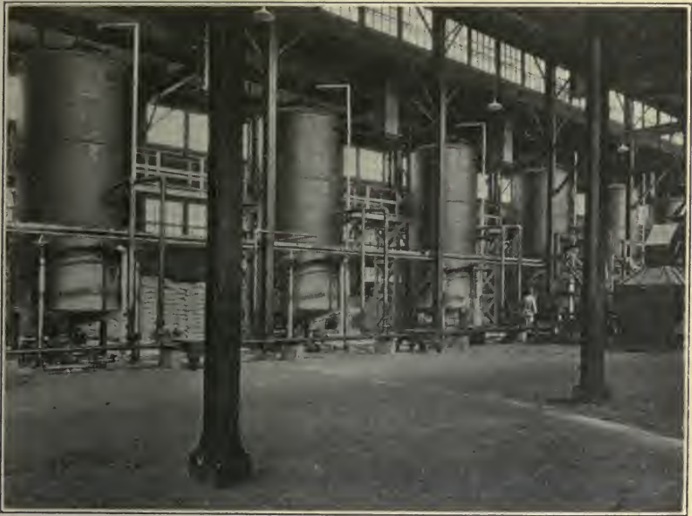
FIG. 27.—Interior of Chloropicrin Plant.
