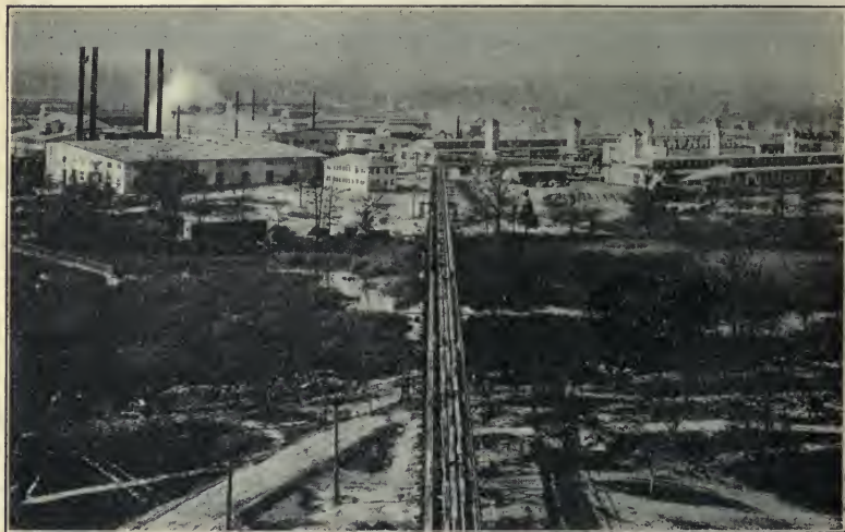
FIG. 19.—Chlorine Plant, Edgewood Arsenal.
