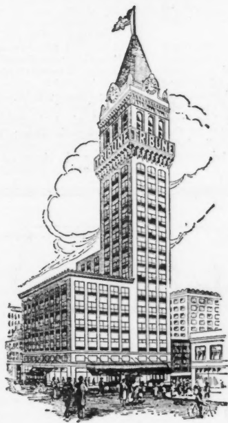
THE TRIBUNE TOWER The 20-Story Addition to The TRIBUNE Building
