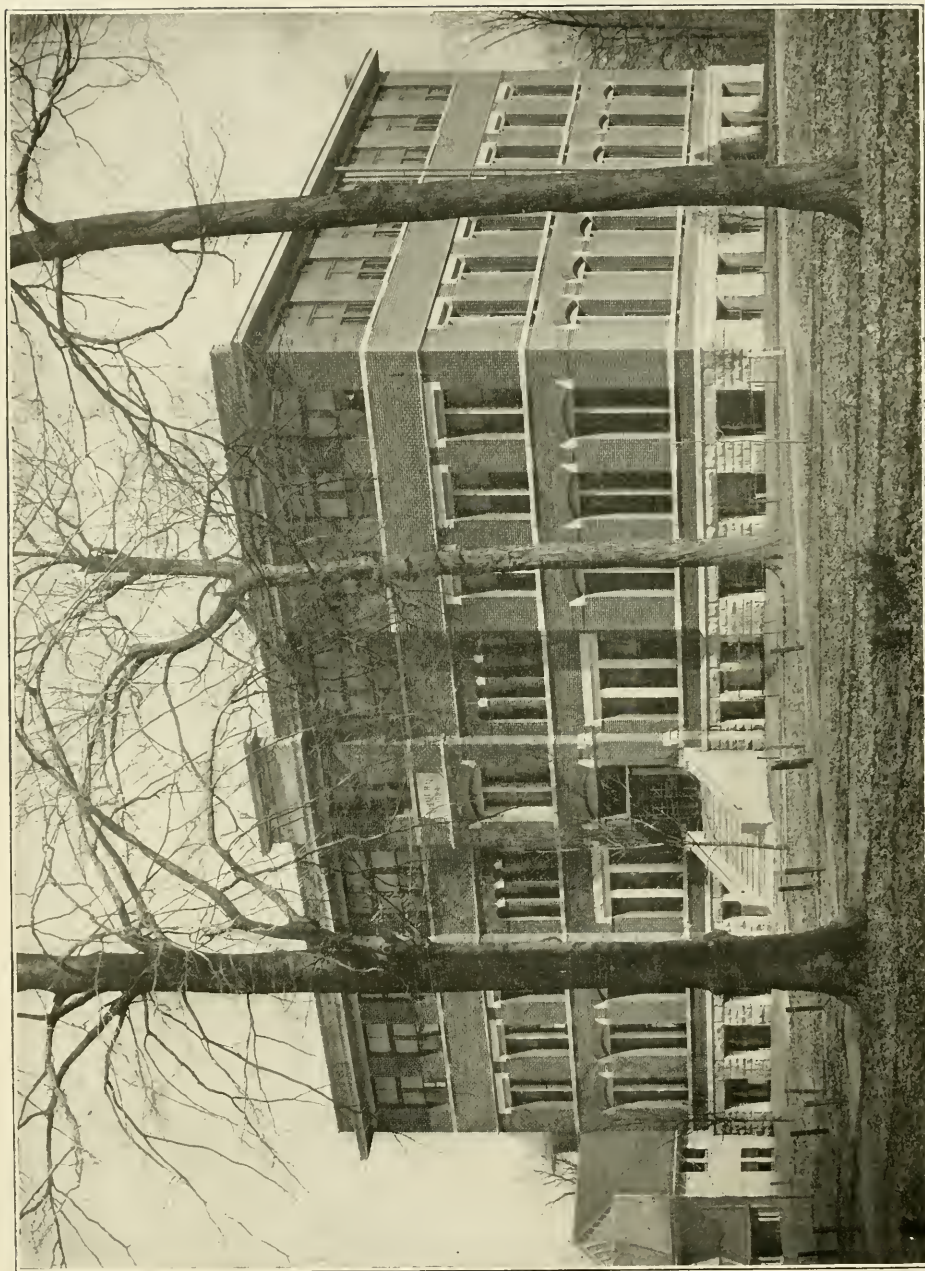
WYLIE HALL (ERECTED 1884) Partially destroyed by fire, 1900; rebuilt with additional story, 1900.
