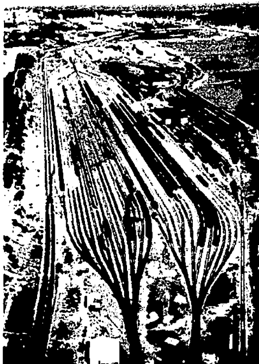
FIGURE 1. Modern automatic hump classification facilities at Lourenco Marques (U/OU)
