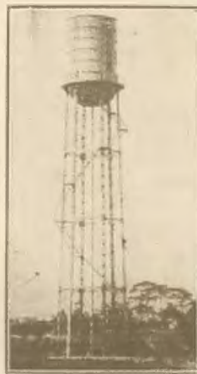
95000 GALLON TANK CANTON WATERWORKS
