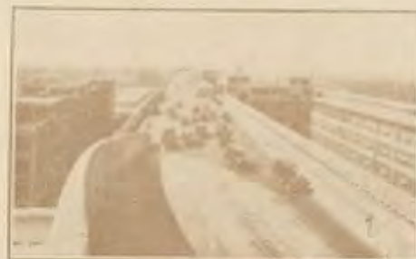
The Roof Track at the LINGOTTO WORKS.
