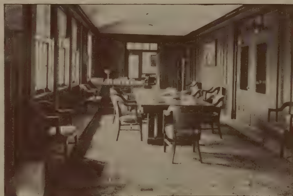
Interior Administration Building
