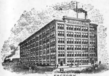
FACTORY 132 ND TO 133 RD ST. & BROOK AVE.
