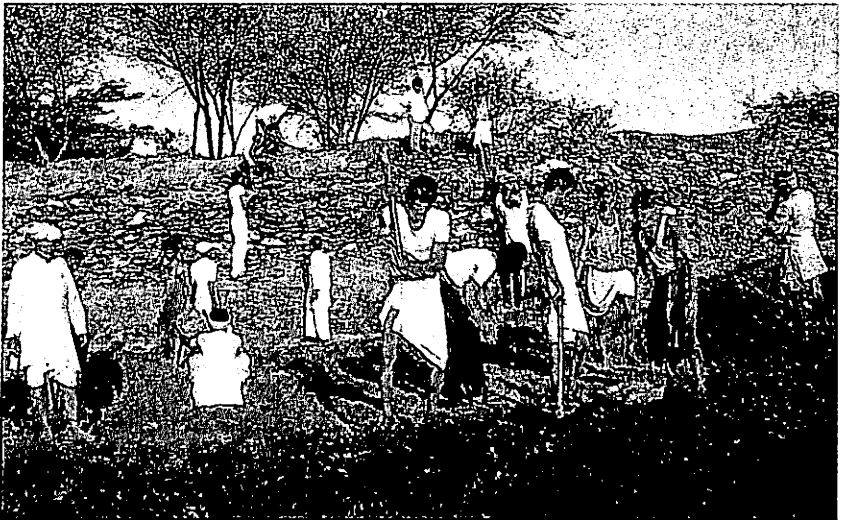
A johad under construction
