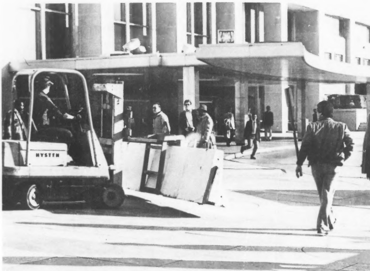
Concrete highway dividers are moved into place. (Photo by Ann Thomas)
