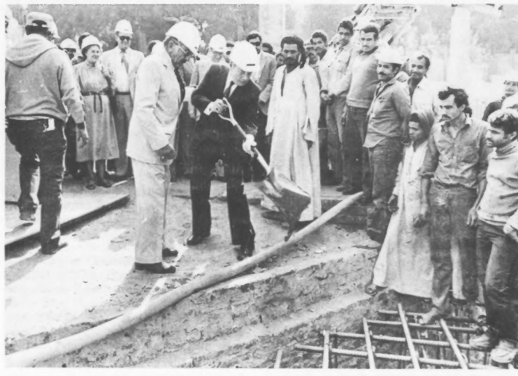
CAIRO, Egypt—Ambassador Alfred L. Atherton Jr. pours first shovel of cement for new chancery office building. With him is Martin Ganon, contractor. Mrs. Atherton is at left.
