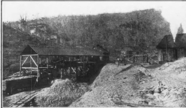
FIG. 5. TIPPLE AT IRON-ORE MINE NEAR ROCKWOOD
