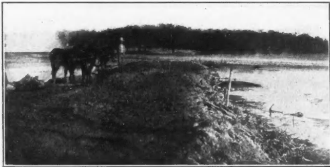
BUILDING DIKES FOR STORAGE OF OIL
