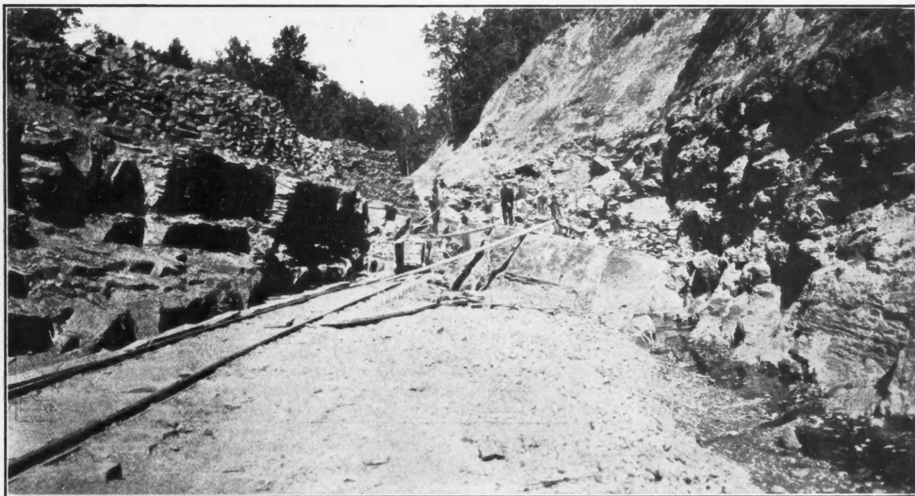
FIG. 1. STRIPPING AT CHAMBERLAIN, OR WELKER, MINE; ORE EXPOSED AT THE SIDES AND AT THE FACE
