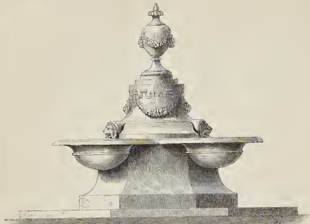
DRINKING-FOUNTAIN IN THE GREEN PARK, LONDON. MR. SYDNEY SMIRKE, R.A. ARCHTGT.
