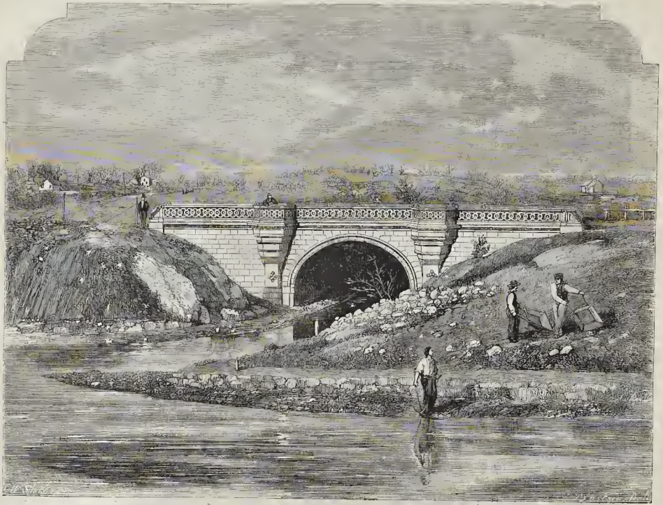
CENTRAL PARK, NEW YORK.— Bridge for Carriage-drive over arm of Lake, near the Raabla. MR. C. VAUX, ARCHITECT; MR. E. C. MILLER, ASSISTANT.
