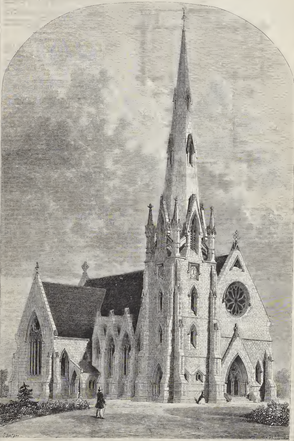
ST. STEPHEN'S CHURCH, SOUTH LAMBETH.—MR. JOHN BARNETT, ARCHITECT.
