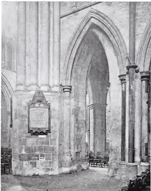
SOUTHWARK CATHEDRAL (LONDON) West Side of North Transept
