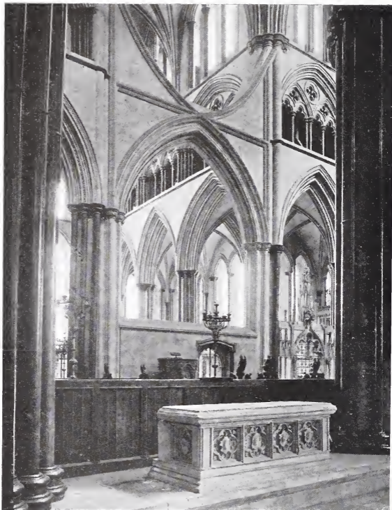
SALISBURY CATHEDRAL Across Choir showing inverted Arch
