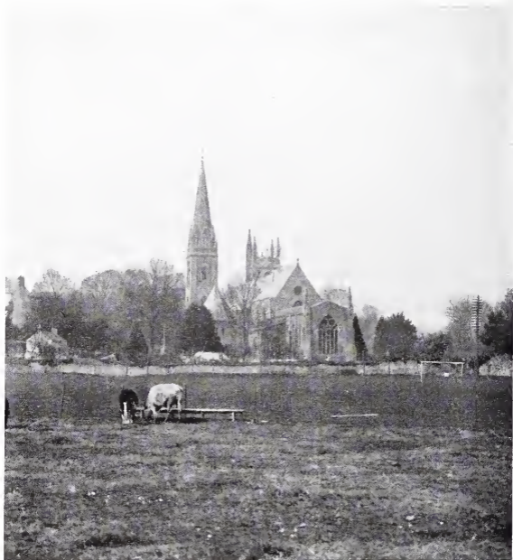
LLANDAFF CATHEDRAL From South-East
