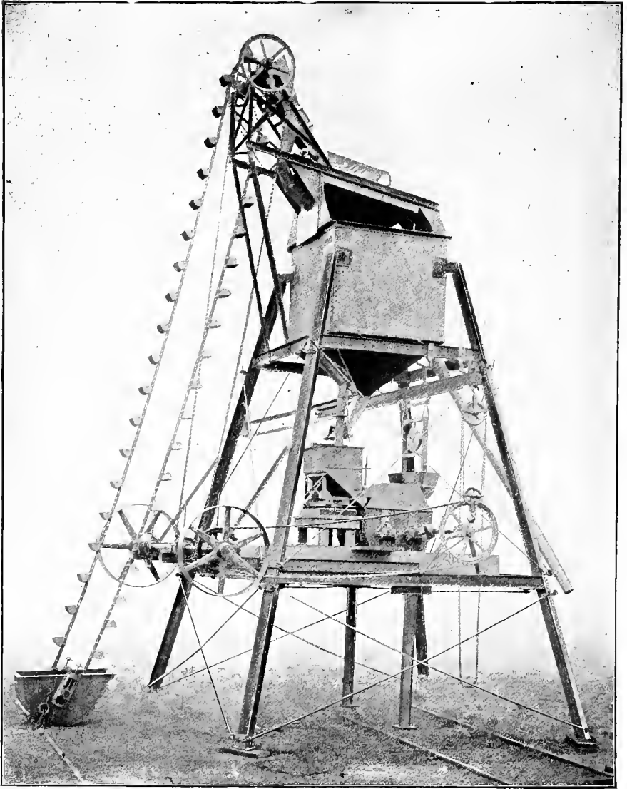
FIG. 22.—Semi-portable Mixing Platform.
