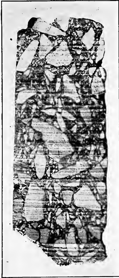
FIG. 14.—Section of Bitulithic Surface, Howard Avenue, New Orleans
