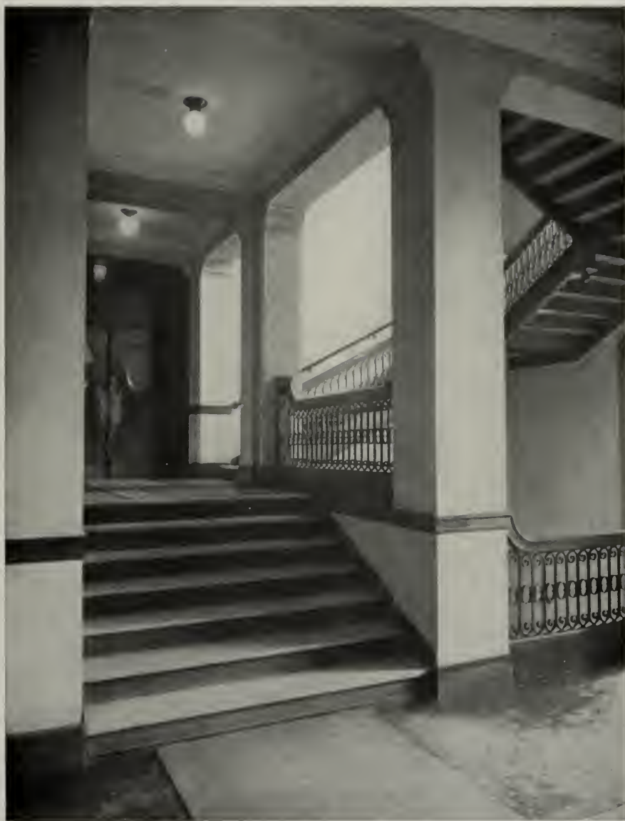
STAIRCASE, SECOND TO THIRD FLOOR, EAST SIDE
