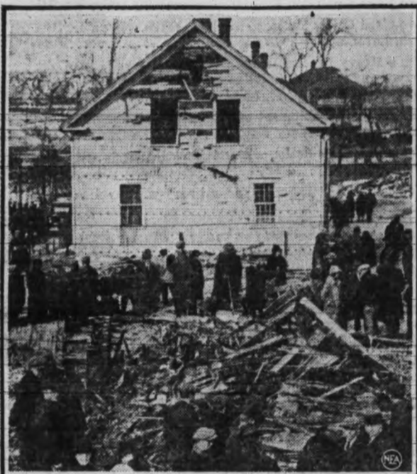
FIFTEEN PERSONS KILLED.—Dynamite used for wood cutting exploded, wrecking two-family home of Michael Conway and Adolard Hamel in Manville, R.I. Fifteen persons lost their lives. In foreground is shown all that remains of the house. Note the rent made in the house next door.
