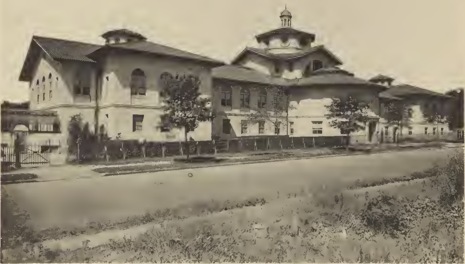
FACADE TOWARD STREET
