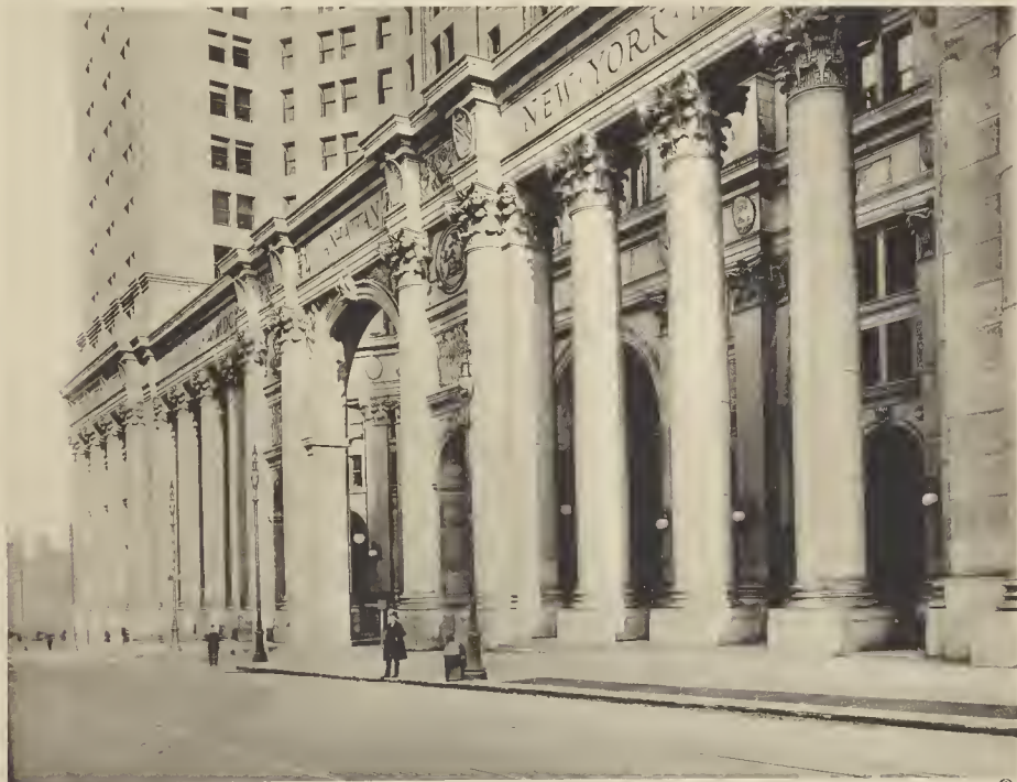
DETAIL OF COLONNADE AT BASE
