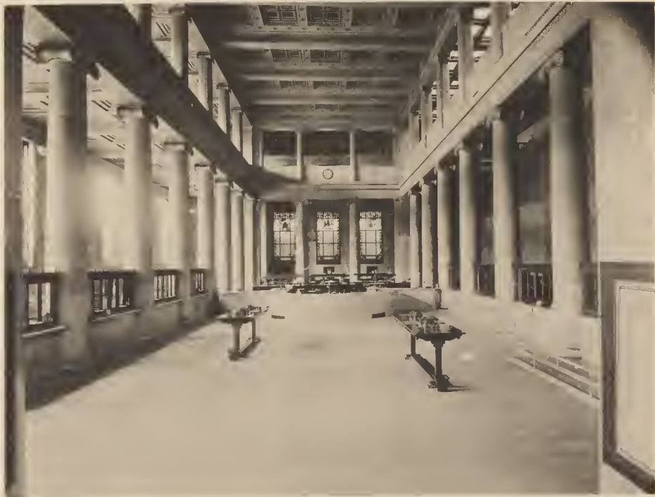
VIEW OF BANKING ROOM
