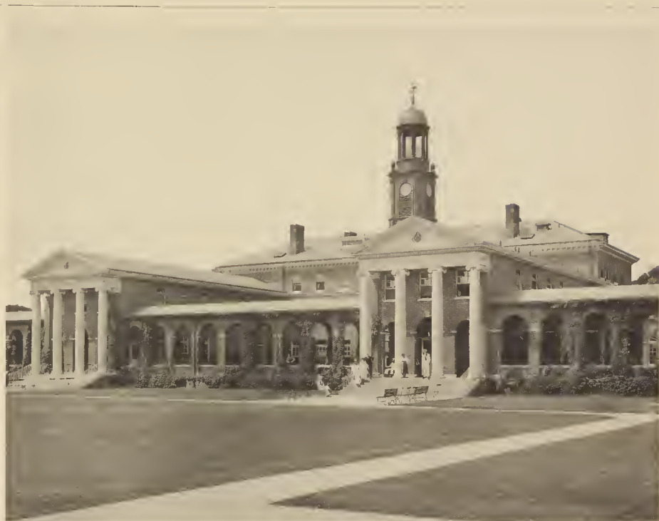
ADMINISTRATION BUILDING, FACADE TOWARD QUADRANGLE
