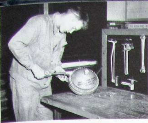
Torque Wrench Application.
