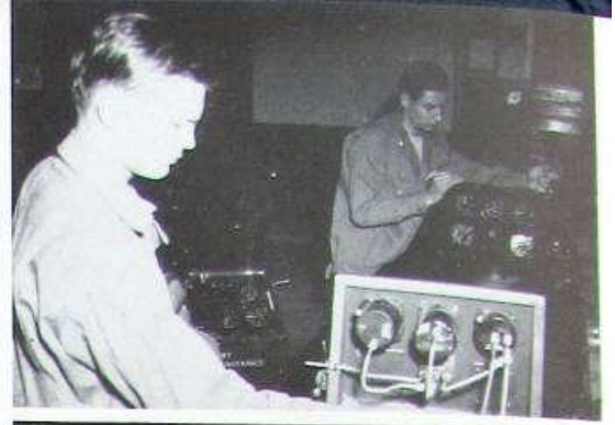
Mockup, Pilot Static System.
