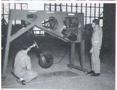
Mockup, Warning and Limit Switches System.
