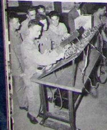
Voltage Regulation Adjustment.
