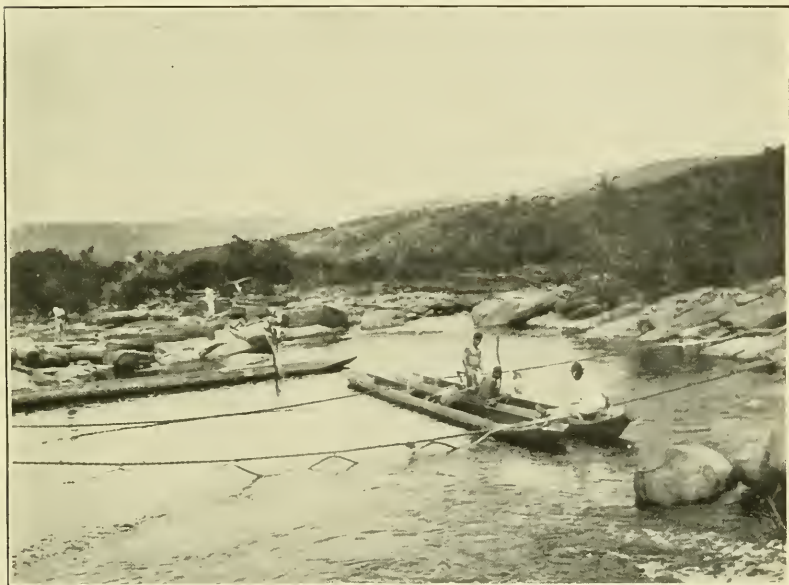
A NATIVE NAKED DIVER PREPARING TO GO DOWN; SUSPENDED FROM THE ROPE IS A TUBE CONVEYING AIR TO A MAN IN DIVING SUIT ALREADY ON BOTTOM.
