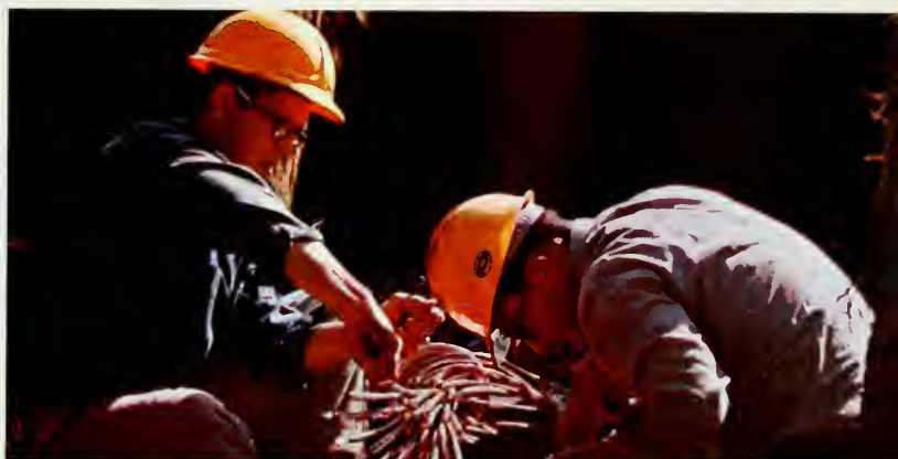
Two-man splicing teams join together the 104 wires and 20 copper tubes of the cable. An average of four splices per mile are needed and are then covered over with a 44-inch lead sheath. Splicing is done in open pits or precast manholes that also hold repeaters.
