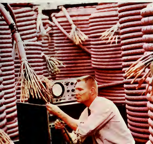
Thirteen units of the Bell System, coordinated by the Long Lines department of AT&T, have joined forces in the cable project. The cable was manufactured at Western Electric's Baltimore Works where, at left, it is being tested to insure dependability.
