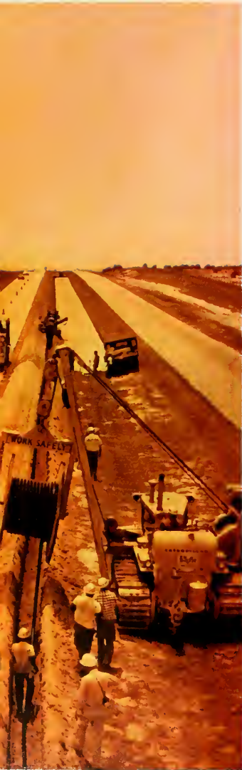
Cable laying techniques vary from the relatively easy going along Florida's Sunshine State Parkway and rich farm land to the rocky terrain of the northeast. Work crews can normally lay two to three miles of cable per day when not faced with unusual soil conditions.
