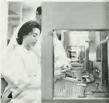
Doors permit devices to pass to work areas in ultra-clean room without contamination.
