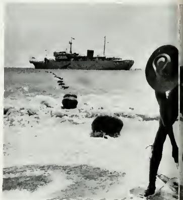
Venezuelan workman removes float from new submarine cable as C.S. Alert stands by.
