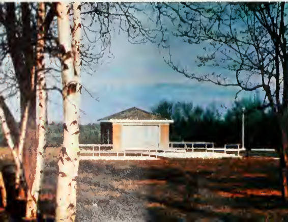
Only portion of the building above ground is garage-like structure through which people enter and leave building.
