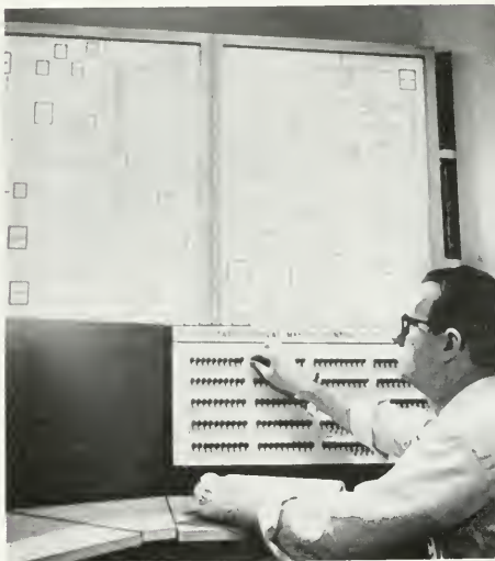
In first Restoration Control Office lights trace outline of simulated circuit failure.
