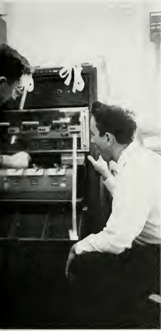
Alfonso Butera of NESC checks out teletypewriter equipment at Suitland, Md., with Donald Posey of Chesapeake and Potomac Tel. Co. Plant. The Bell System's teletypewriter network ties together the various stations of ESSA, ranging from points in Virginia to Alaska.
