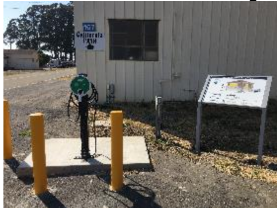
Figure 14: Aerovironment Level 2 Charger
