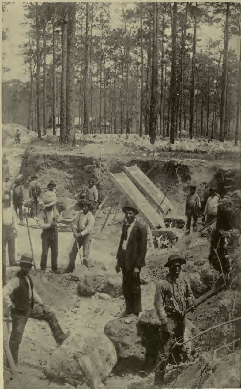
FORIDAL ROCK-PHOSPHATE MINING. Working in "boulder" material after removal of top soil.
