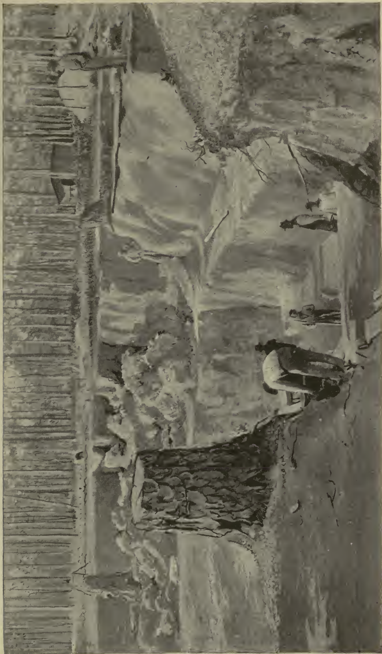
FLORIDA ROCK-PHOSPHATE MINING. Extracting "boulder" material from matrix of sand and clay, Empire State Company's mines, Citrus Co.
