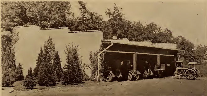
The Garage at Chase.
