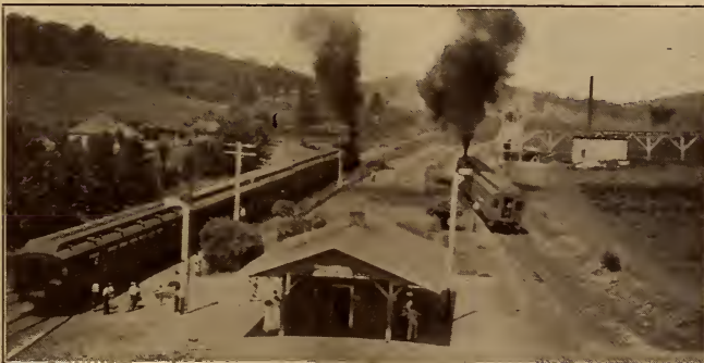
The City of Chase is Entirely Surrounded by Railroads. We Get Action Here on Express Shipments.
