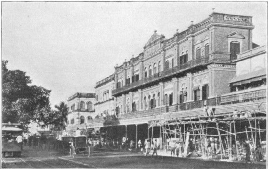
Das Grand Hotel am Tschoringhi in Kalkutta.
