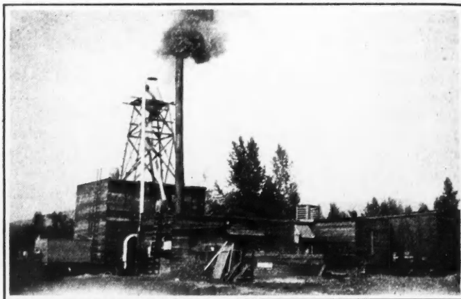
Treatment plant at Libby
