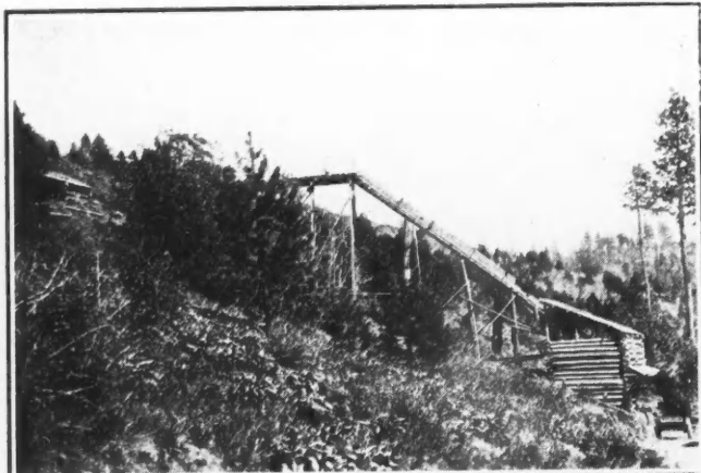
End of tramway from mine, and chute to ore bins
