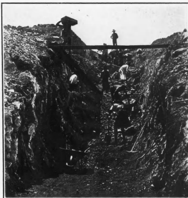
Native workmen cleaning out one of the ancient excavations at the Star of the Congo, preparatory to starting modern mining methods.
