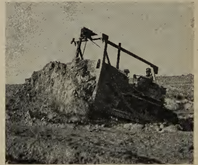
Excavating for a pond.
