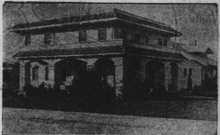
Home of L. H. Wilson, 204 W. Milford—Corner Milford and Orange
