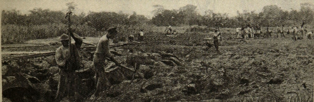
Trinidad Lake, showing asphalt dug for Genasco Ready Roofing.
