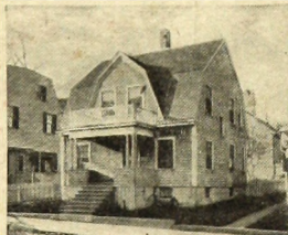
A No. 22 IDEAL Boiler and 240 ft. of 38-in. AMERICAN Radiators, costing the owner $115, were used to Hot-Water heat this cottage.
