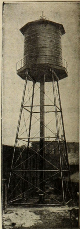
Erected for LIBBY GLASS CO., TOLEDO, OHIO.
