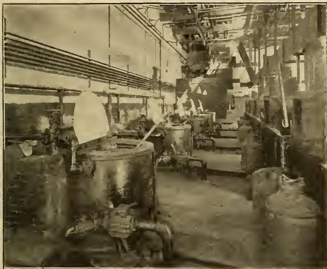
Fig. 22. Centrifugal drying machines for removing all traces of moisture from the cotton.
