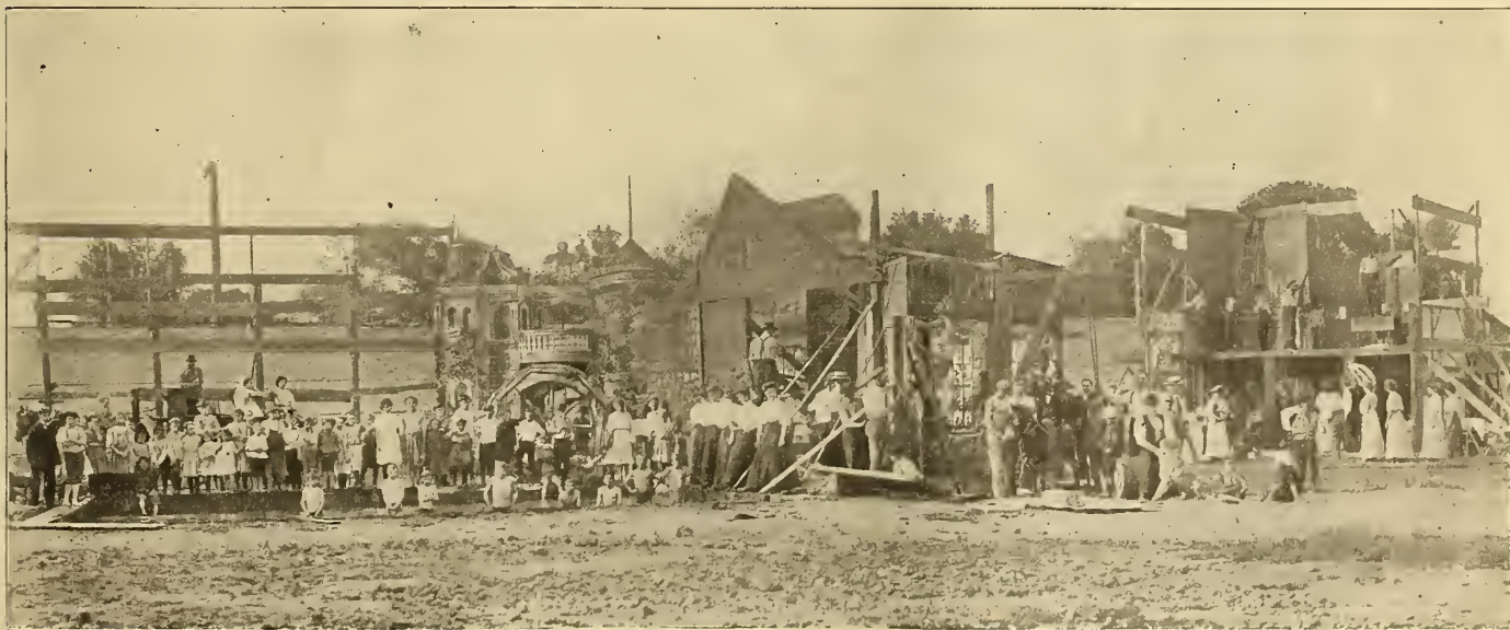
Fig. 32. Taking a "yard" scene in the rear of a film manufacturers' studio. The nature of the buildings and scenery may be seen at the right. The "tank" used in producing aquatic scenes is in the middle foreground at the left.
