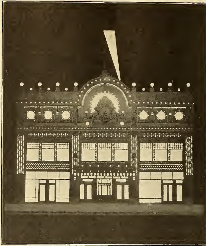
How New Isis Theater Will Be Illuminated with Four Thousand Incandescent Lamps, Varying from Four to Fifty Candlepower.
