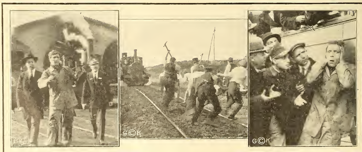
Scene from "The Rival Engineers." Copyrighted 1913 by George Kleine.
