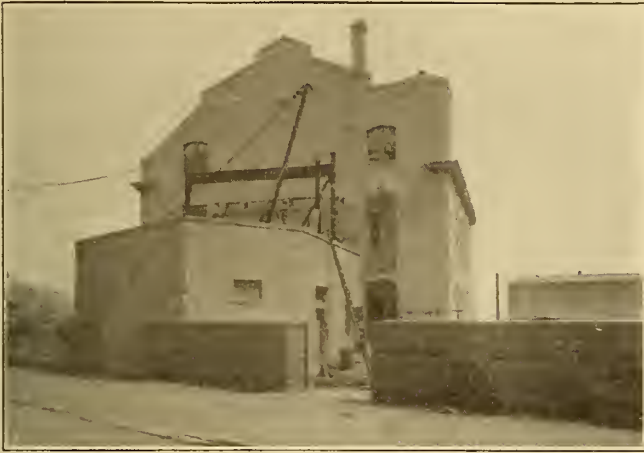
View of Pathe Studio Looking East.
