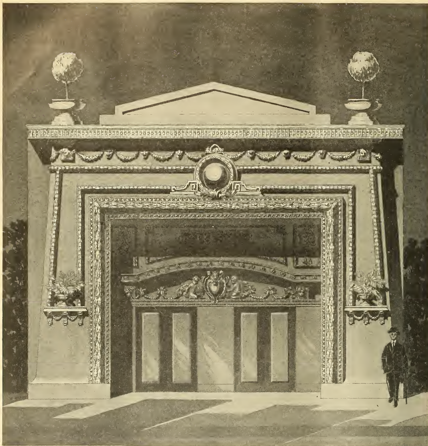
Edmonton Theater, Edmonton, Alberta. Front Designed by Decorators' Supply Co.
