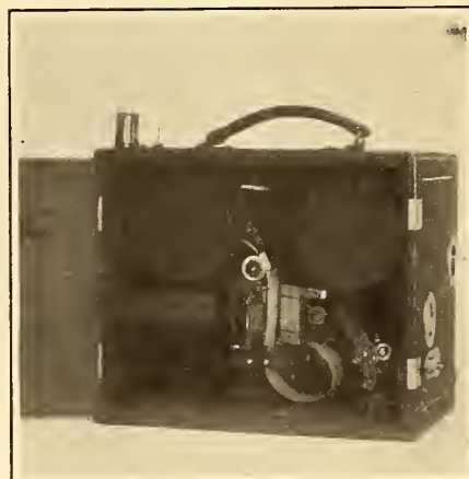
Fig. 6.—Interior View Showing Mechanism and Paper Negative in Position in Opened Gate.
