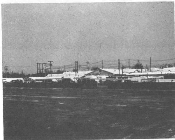
Helicopter Pad at NSA Danang. Note Triage areas in quonset hut structures and hospital in background.
