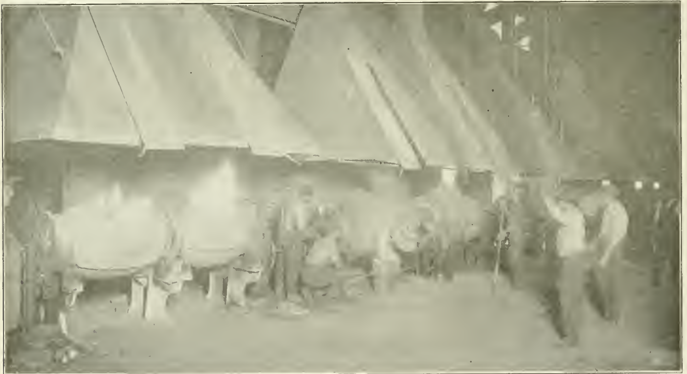
Tilting Furnace in a Bronze Foundry
