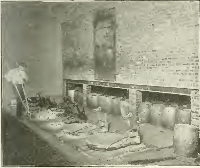
Pit Furnaces Operated with Oil and Gas.
