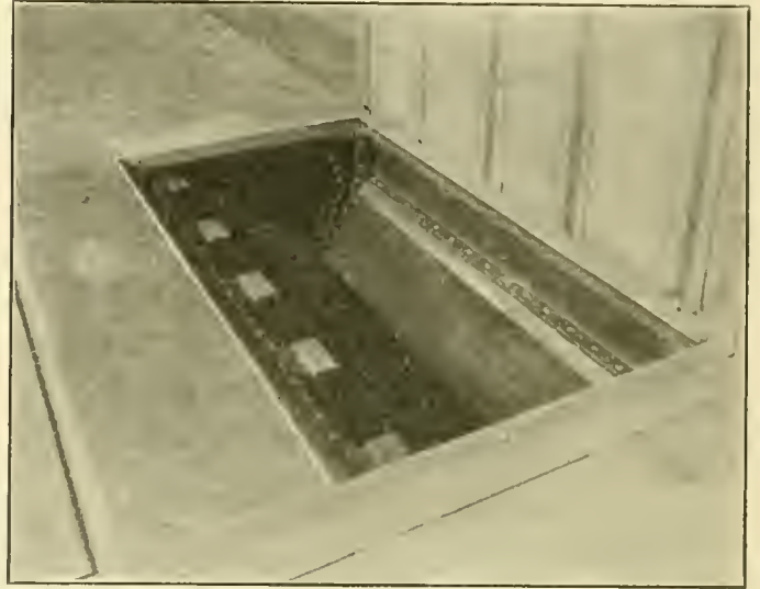
Floor Section Raised for Grain Loading
