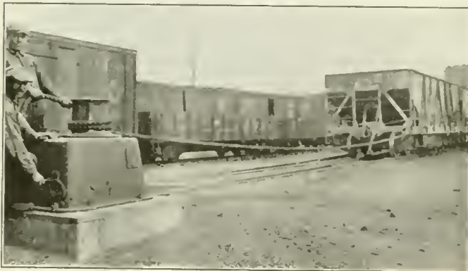
Hauling a Cut of Cars with the Electric Winch
