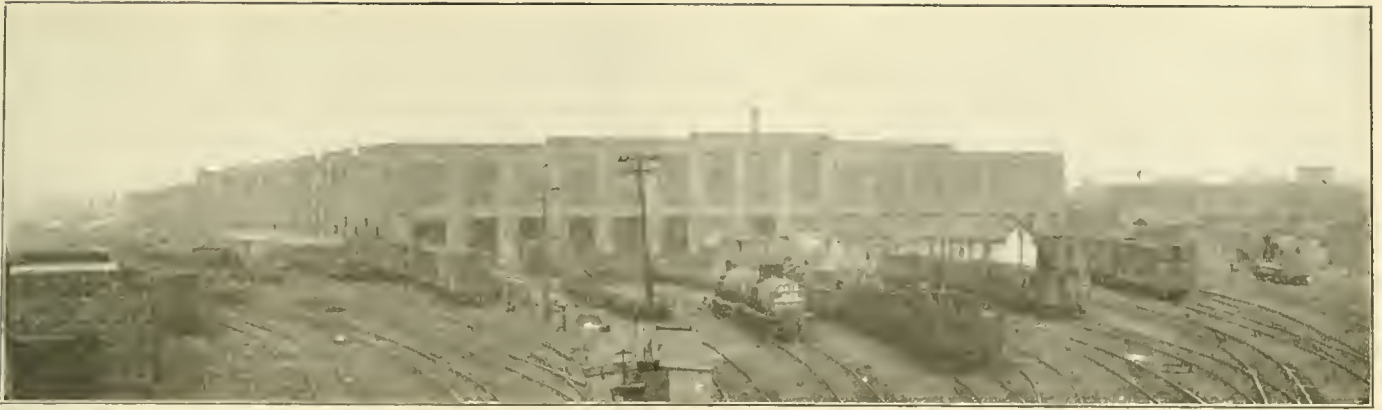
General View of the East Buffalo Car Shop
