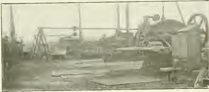
Fig. 10—Part of the Equipment for Handling Steel Car Work
