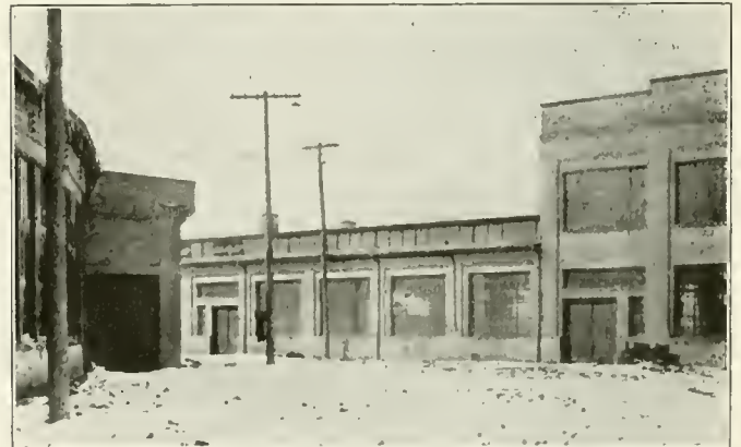
Relation of the Drop Pit Extension of the Roundhouse to the Back Shop
