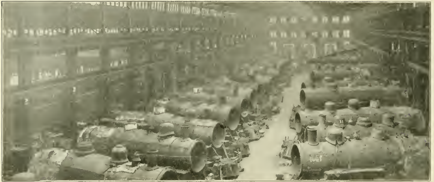
Looking Down the Erecting Bay in Silvis Shop
