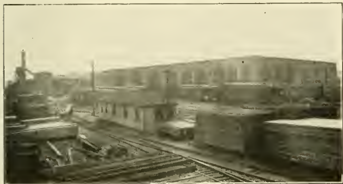
North End of the Erecting Shop, Planing Mill at the Left
