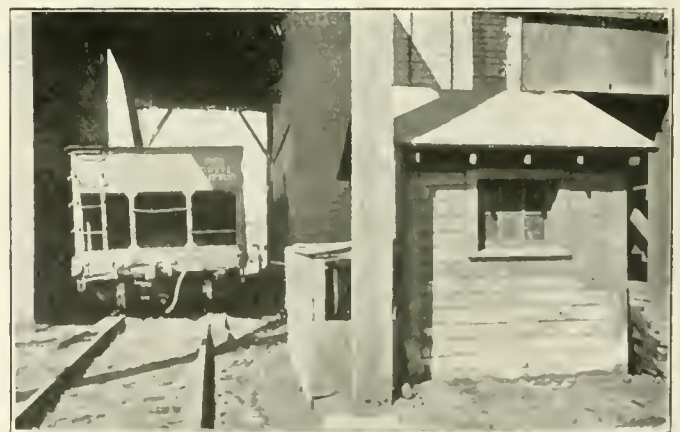
Fig. 2. Car Hauling Winch Installed at Coaling Station
