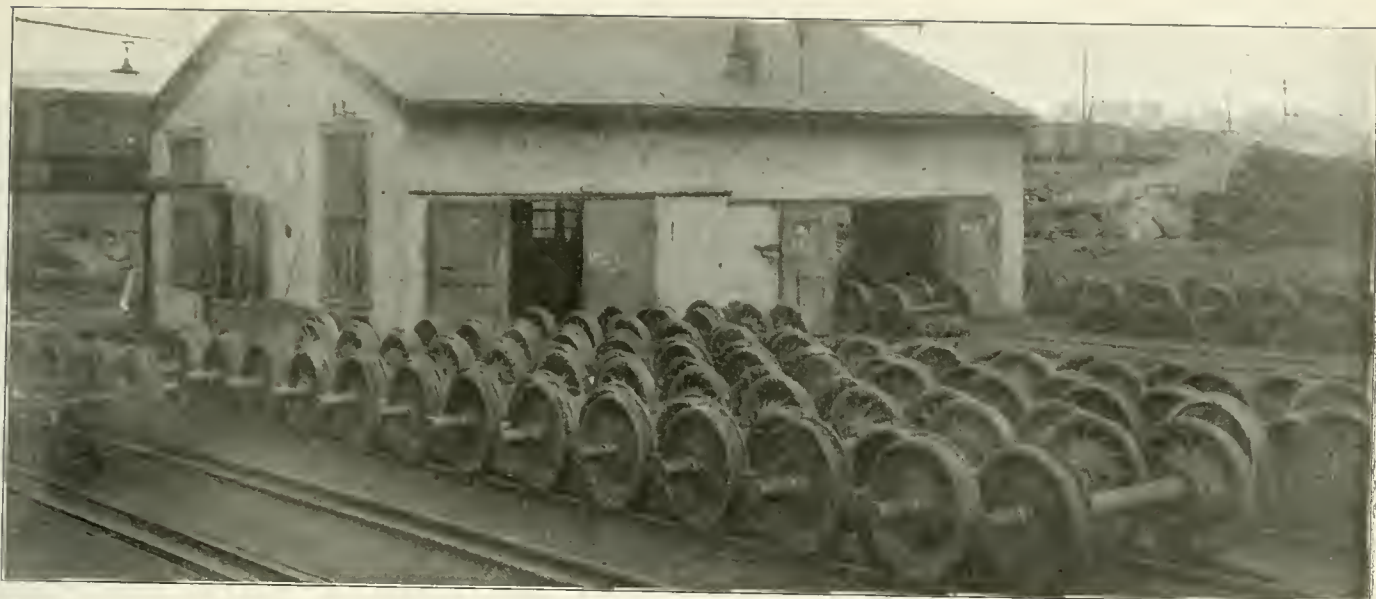
View of Inspection Shed and Accumulated Car Wheels
