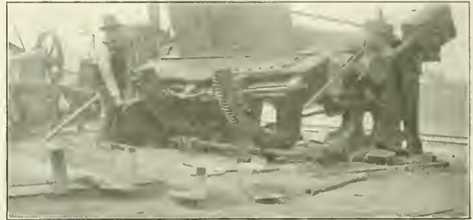
Fig. 5—Flanging a Floor Sheet In the Power Brake
