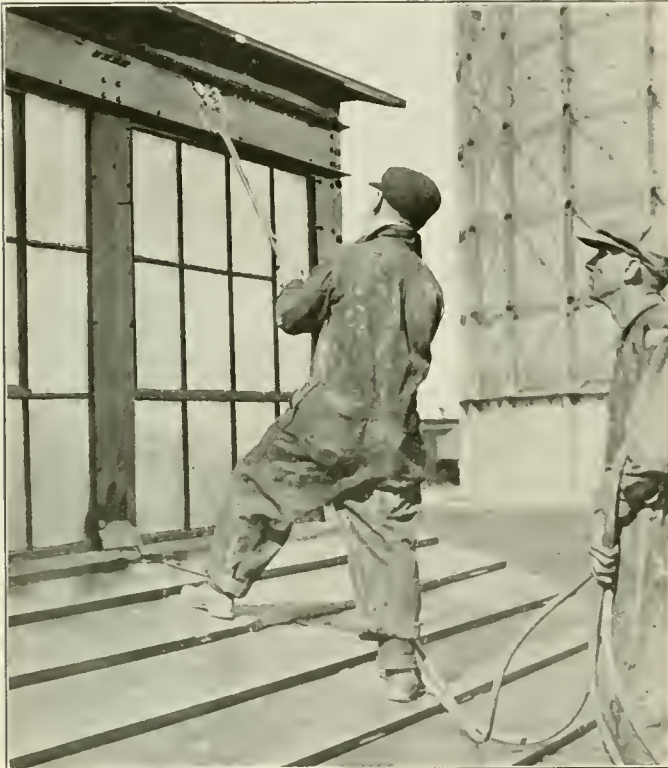
Vortex Painter in Use On Metal Building
