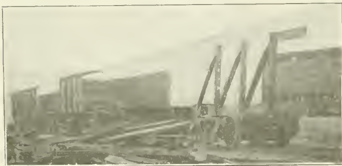
Fig. 11—Steel Cars Dismantled for Repairing
