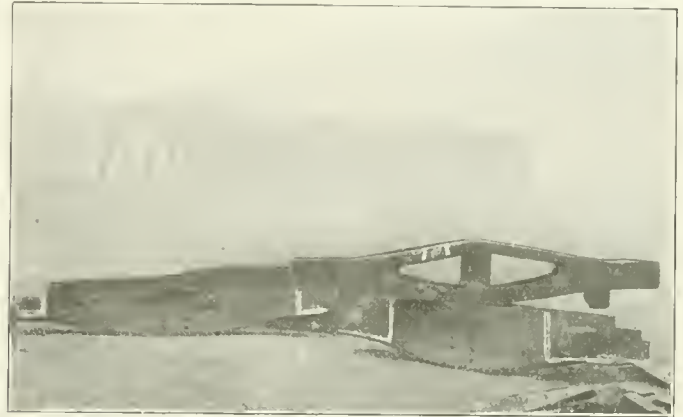
Fig. 9—Defective Bolsters Prepared for Welding
