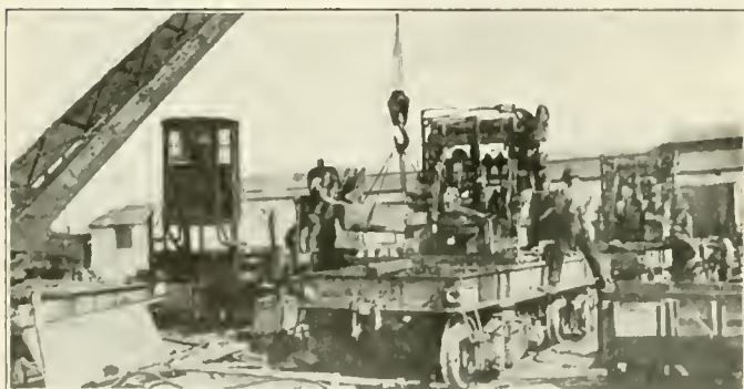
Erecting Locomotive Cranes
