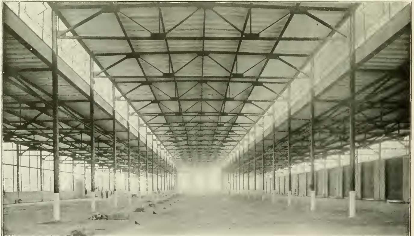
Interior View of the Transverse Shop
