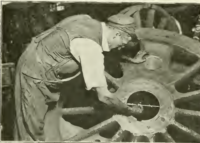
Fig. 4.—Calipering the Bore of a Wheel Center.
