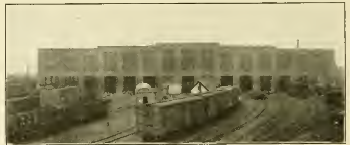
South End of New Steel Shop
