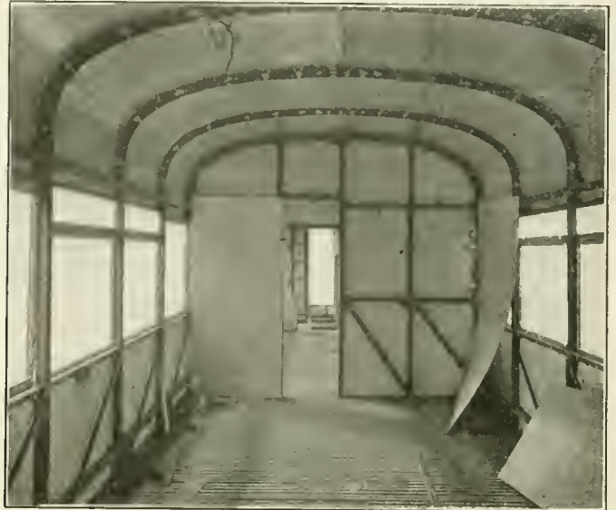
Interior View of Motor Car During Construction
