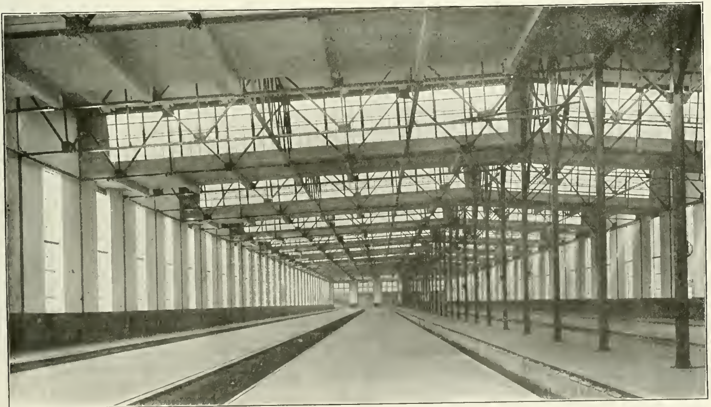
Interior of the Longitudinal Type Shop
