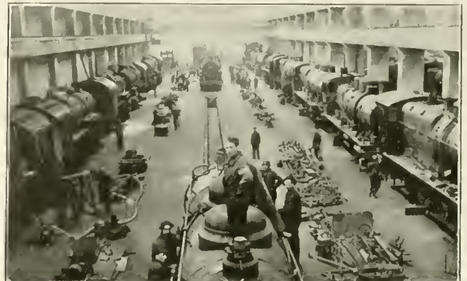
One of the Two Bays of the Erecting Shop of the A. E. F. Engineers at Nevers, France. American Locomotives on the Left and Centre Tracks. French Locomotives on the Right Hand Track.
