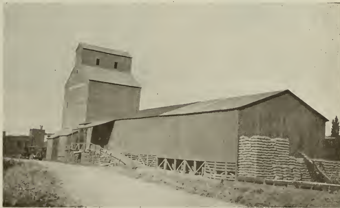
ELEVATOR OF THE EDWALL WAREHOUSE COMPANY, EDWALL, WASH.
