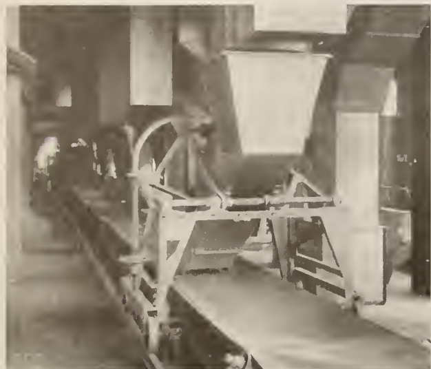
VIEW IN ONE OF THE CONVEYOR GALLERIES
