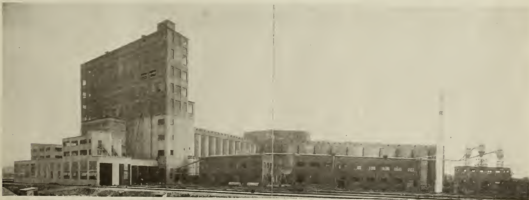
THE SANTA FE ELEVATOR "A" AT ARGENTINE, KANSAS CITY, KAN., SHOWING RECENT ADDITION TO OLD PLANT
