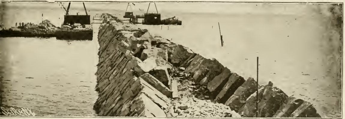
STONE BREAKWATER, SHOWING TOP ANGLE STONES.
