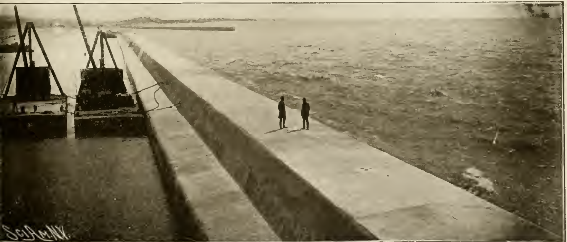
THE COMPLETED CONCRETE BREAKWATER.
