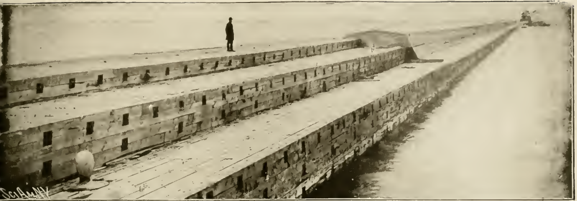
ORIGINAL CRIB SUPERSTRUCTURE IN FOREGROUND; CONCRETE RECONSTRUCTION IN DISTANCE.
