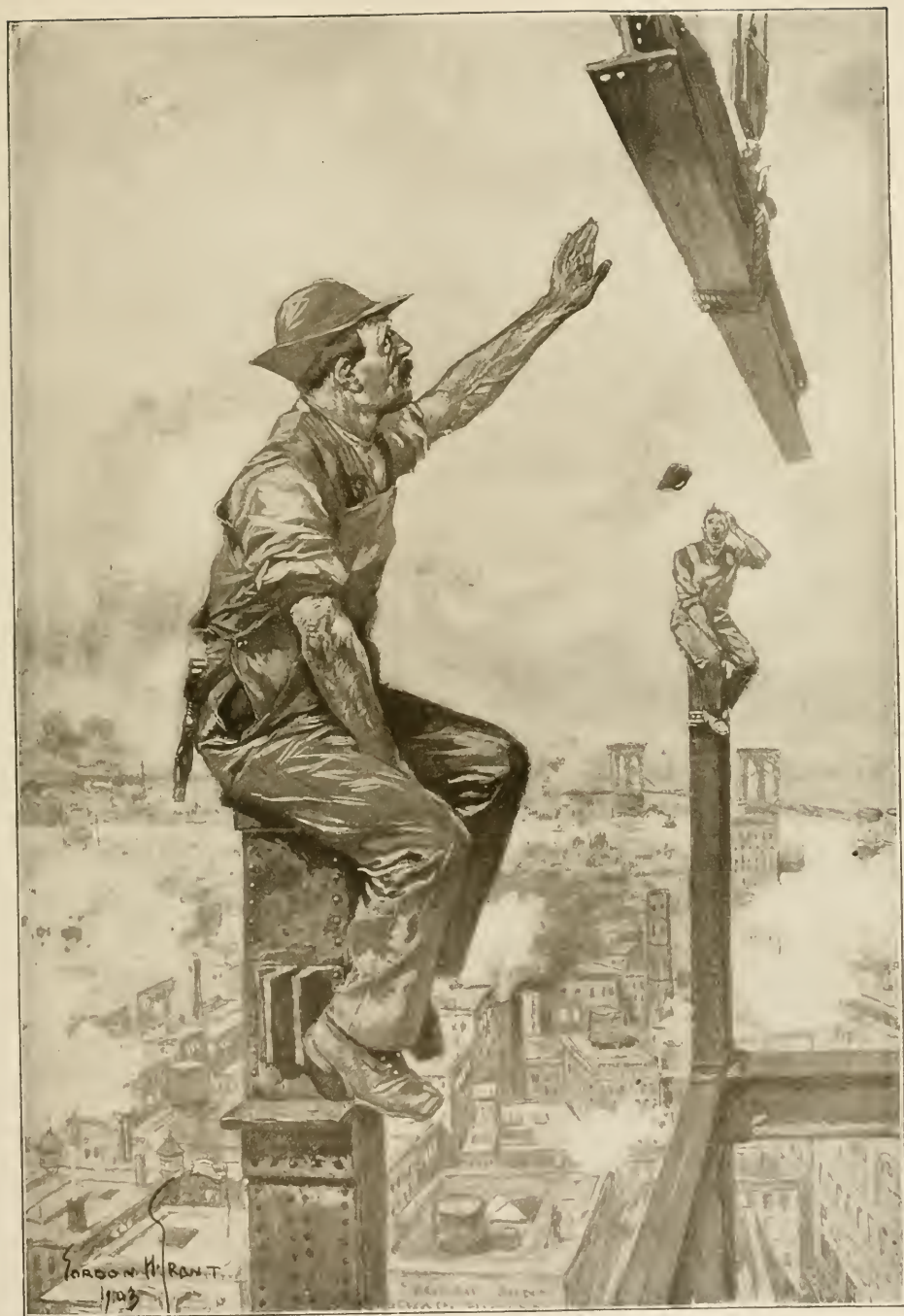
STEEL SKELETON CONSTRUCTION.
