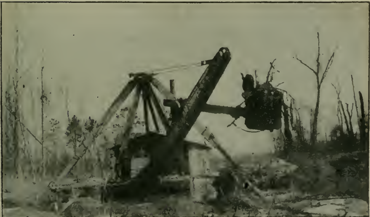
FIG. 2.—DREDGE DIGGING DRAINAGE DITCH THROUGH A SWAMP.
