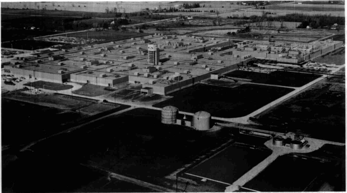
Figure 1 - Ford Motor Co. - St. Thomas Assembly Plant-Waste Treatment Plant in right foreground.
