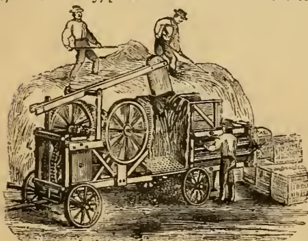
Fig. 1.—DERICK & CO.'S HAY-PRESS.
