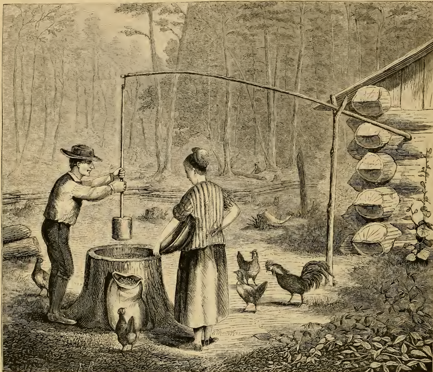
A SETTLER'S PLUMPING MILL.—DRAWN BY R. E. ROBINSON.—Engraved for the American Agriculturist.
