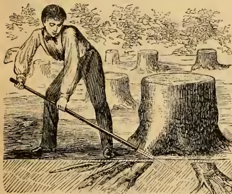
Fig. 2.—BLASTING WITHOUT BORING.
