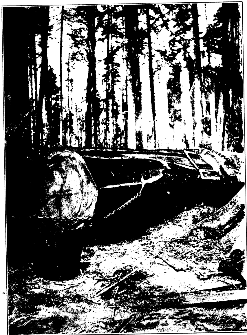
LOGS HAULED BY "DONKEY" ENGINE AND CABLE, SHOWING METHOD OF "HOOKING ON," CRESCENT CITY, CAL.
