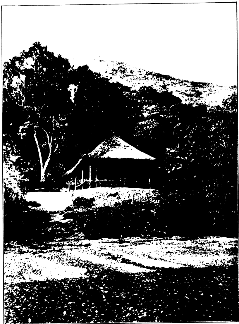
SPRING WHICH SUPPLIES THE TOWN OF CULION WITH WATER—GENERAL VIEW.
