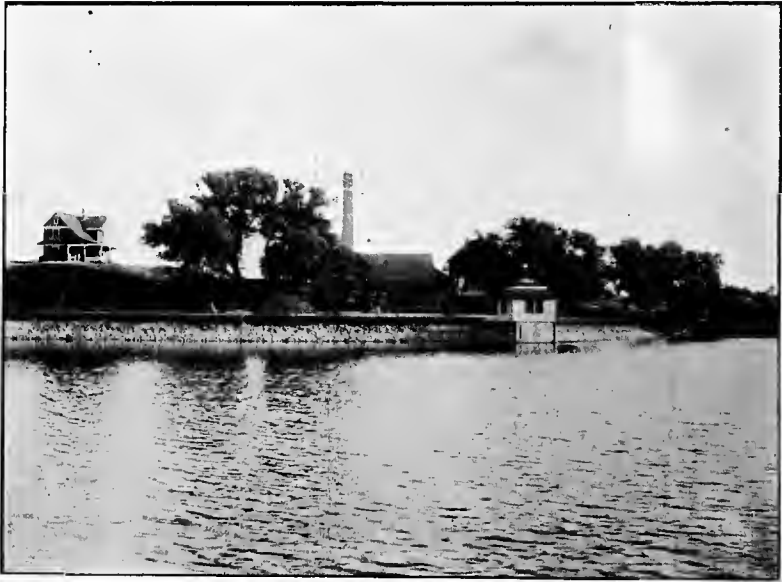
Beverly Pumping Station.
