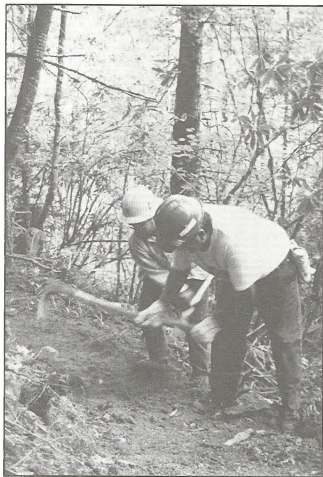
Trail construction on the Eugene District - Photo by Doug Huntington.
