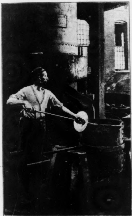
Fig. 3.—Testing Temperature of a Ladle of Molten Iron With Angle Pyrometer.
