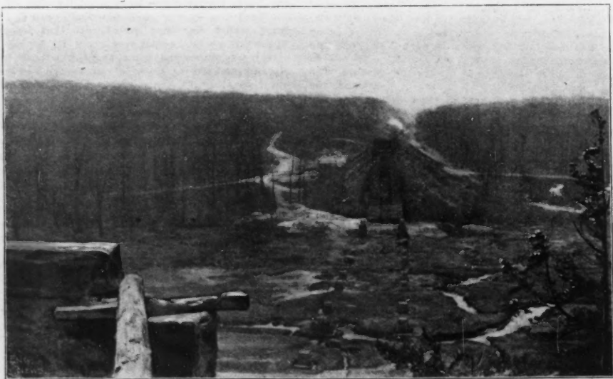
FIG 2.—VIEW OF VIADUCT SITE SHOWING PIER AND "FLOW" OF EMBANKMENT FILLING.
