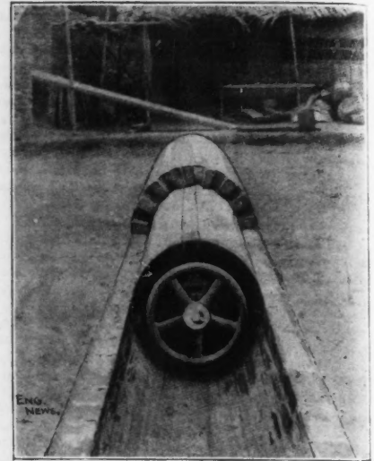
Fig. 1.—A Collapsible Center for Sewer Construction. Burns & Co., Ltd., Calcutta, India, Makers.
